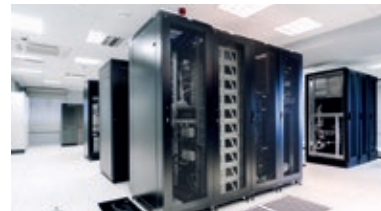
Connection of generators for a server room UPS (New Zealand). Series TH405.
