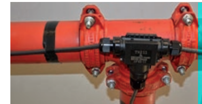
Connection of heating cables (Italy). Series TH211.
